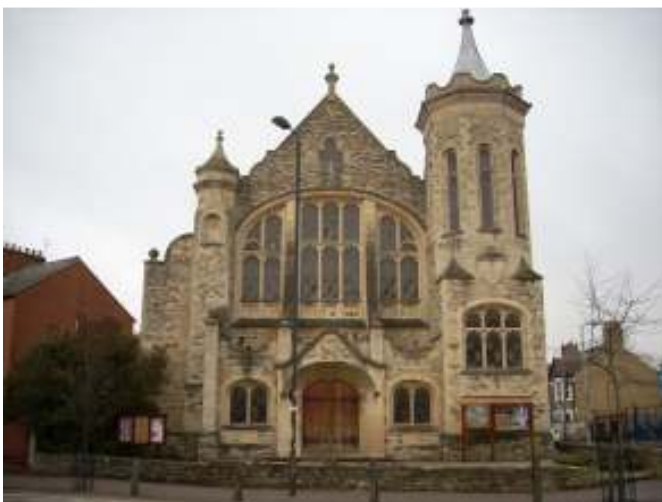
Cowley Road Methodist Church, Oxford (Grade II listed 28 Jun 72, SP 5205 19/706)
