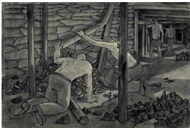
Miners repairing bad roof (watercolour on paper)
